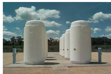
Typical SNF Storage Casks
